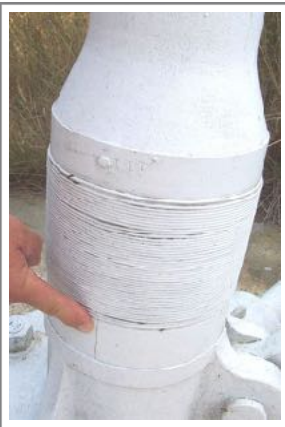
Martin Knudsen's repair of the rear range light.
