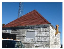
The paint shed shingles were removed and new shingles purchased by USFWS. FOPPI paid for the labor to re-shingle the pain shed roof.
