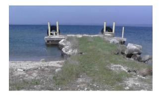
Time, high lake levels and storms seriously damaged the last 40 feet of the pier, the last 25 feet of the west break wall and the ferry haul road along the northeast side of Plum Island.
