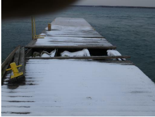
Sections of the dock popped out in a winter storm. Section rebuilt by Iron Works Construction .
