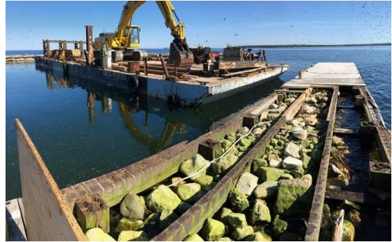
Sections of the dock popped out in a winter storm. Section rebuilt by Iron Works Construction .
