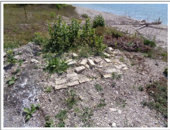
Plum Island front range light remnants, 2021. Photo by Eric Bonow.
