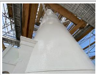
The rear range light with fresh paint and surrounded by scaffolding.
