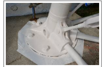
Repainted support post.
