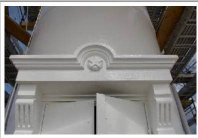
Architrave above the range light doors.
