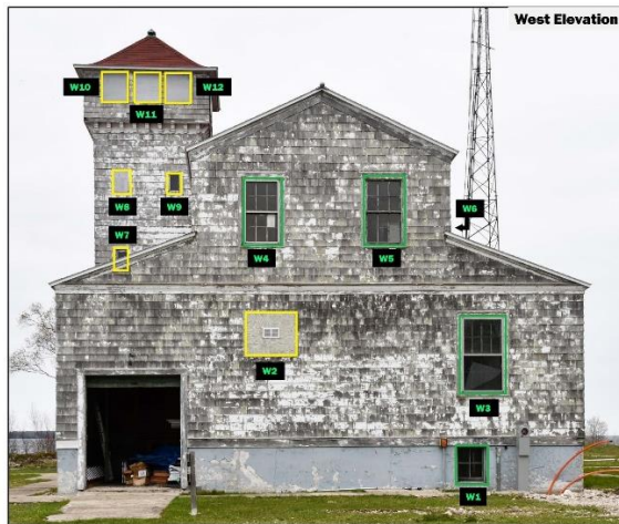
Plum Island Life-Saving Station Crew Quarters Window Survey, June 2019
