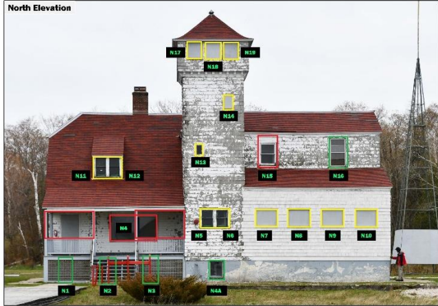
Plum Island Life-Saving Station Crew Quarters Window Survey, June 2019
