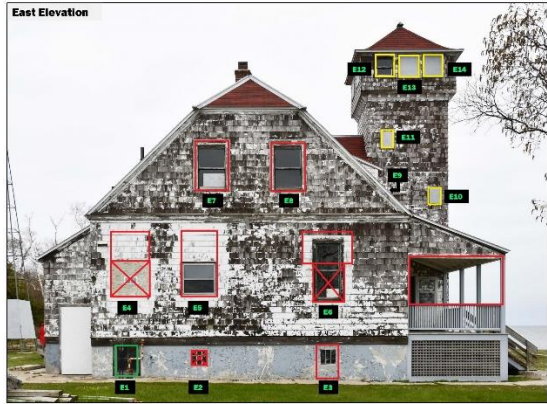
Plum Island Life-Saving Station Crew Quarters Window Survey, June 2019
