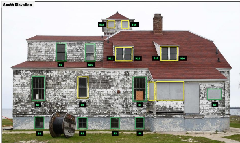
Plum Island Life-Saving Station Crew Quarters Window Survey, June 2019
