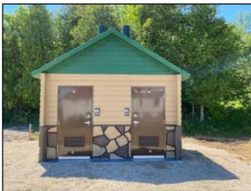
Vault toilet on Plum Island
