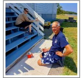
Kimberly and Dallas putting on a second coat of paint.
