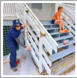
Kimberly and Ginnie scrape the porch railing in preparation for painting.
