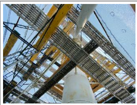
A view of the range light from under the shroud.
