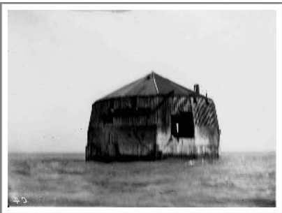
North Point second intake crib structure. Photo courtesy of Milwaukee Water Works.
