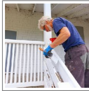
Paul putting on the first coat of white paint.
