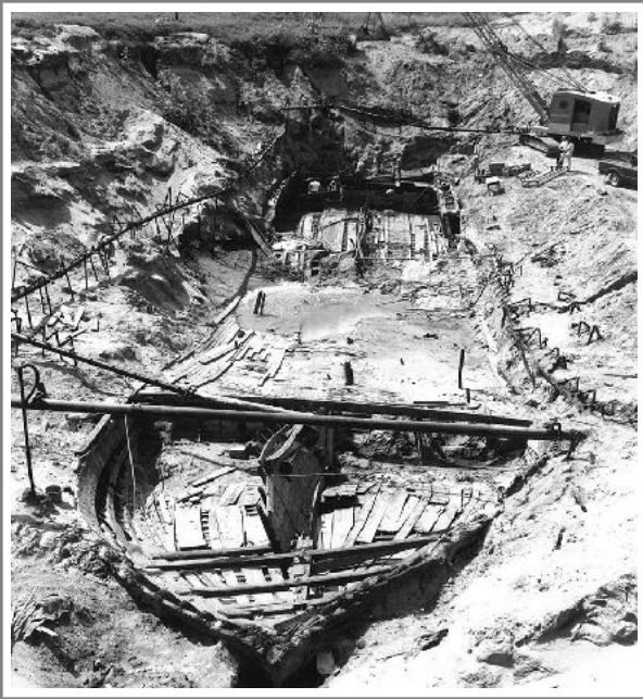
Excavation of the Bertrand .
