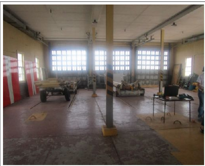
The boathouse in its current condition.
