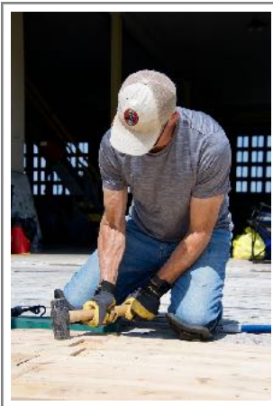
Stiles taps boards into place.
